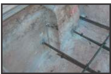
Renforcement du joint
