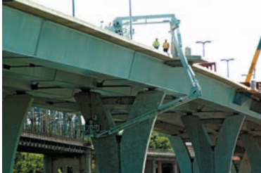
Edge of Bridge
