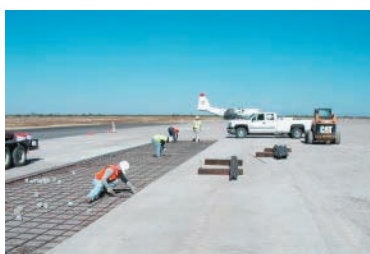
Slab connections
